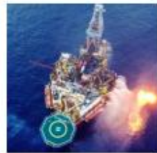
PV DRILLING VI (JU) Year: 2015
