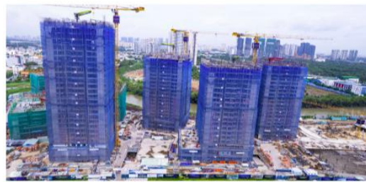
TOWER 5,7: 20 TH FLOOR WORK TOWER 6: 19 TH FLOOR WORK TOWER 8: 26 TH FLOOR WORK UNDER CONSTRUCTION PROGRESS
